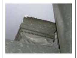
Shows air leakage around gap in ceiling and duct return. Caulk or use expanding foam around seam for a better seal.
