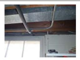
The following photos are examples of utility penetrations and framing gaps in the foundation and rim joist of the home. All gaps should be airsealed with caulk or foam, then the rim joist should be insulated to R10 using rigid foam board with all seams sealed with caulk.
