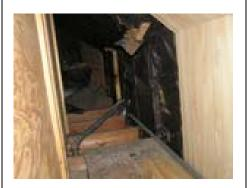
Side attics appear to be uninsulated. Add insulation in floor spaces in side attics where accessible.
