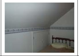
East dormer wall lacking insulation; could be blown from interior.
