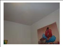
Location of removed chimney is cold. This chaseway may still be open the peak attic and cold air from attic is settling above this ceiling. Look for gaps at the attic floor above here to seal with caulk or foam.
