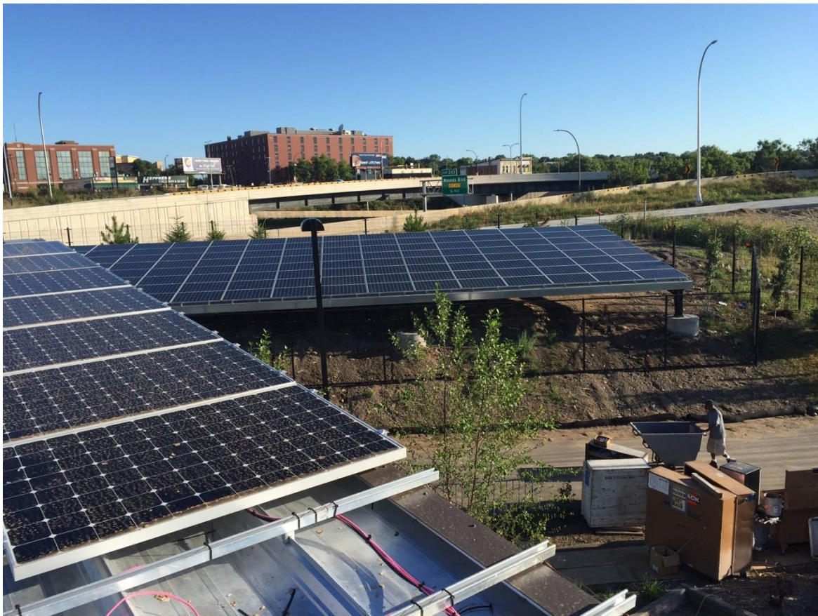
Image 8. Northeast array solar panel installation; August 10, 2015
