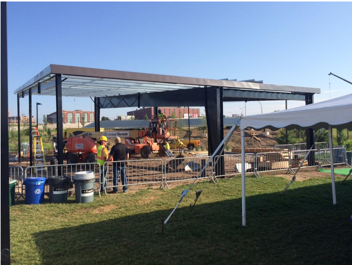
Image 4. Pavilion array framework; June 26, 2015
