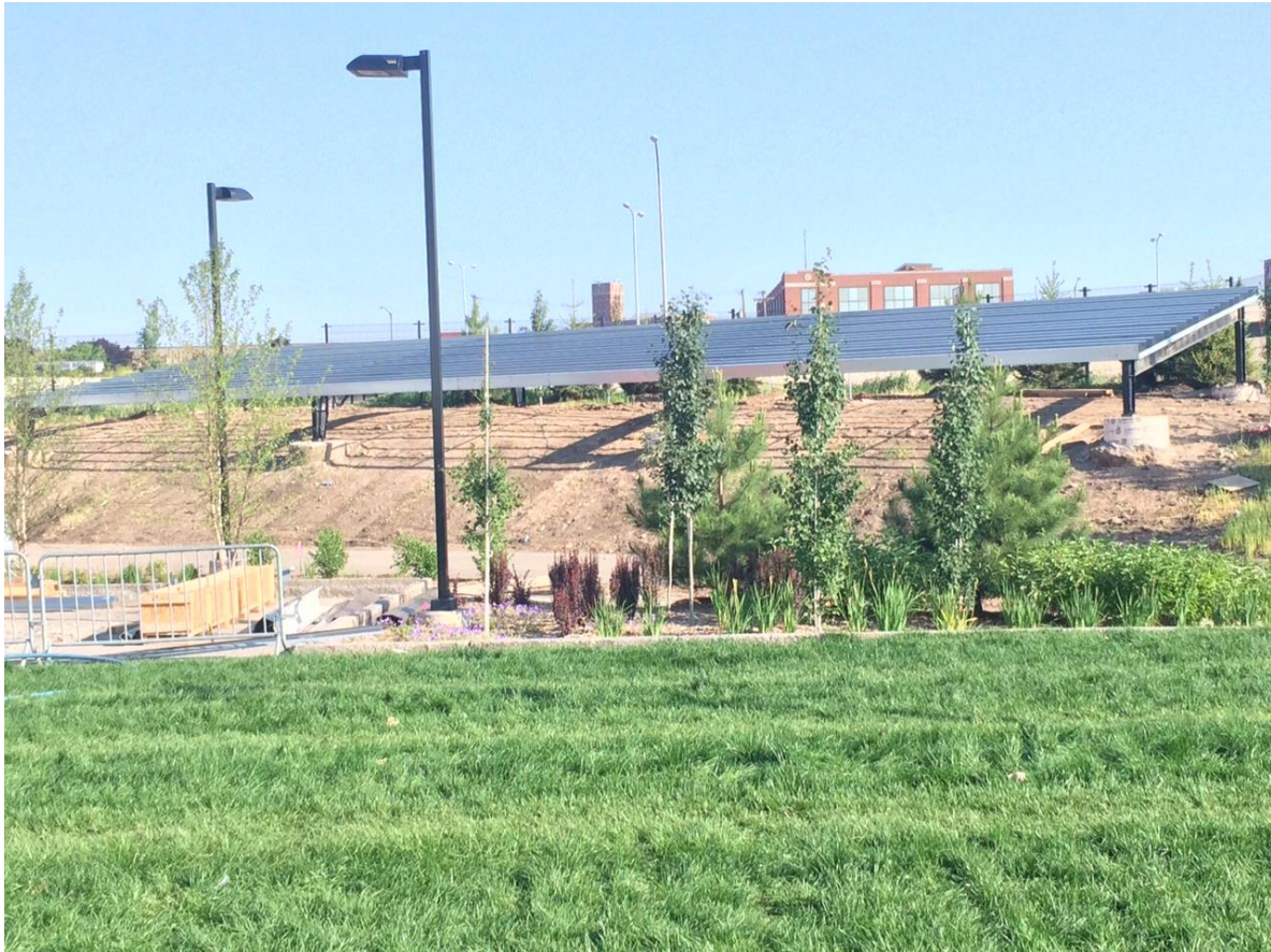
Image 3. Northeast array framework; June 26, 2015
