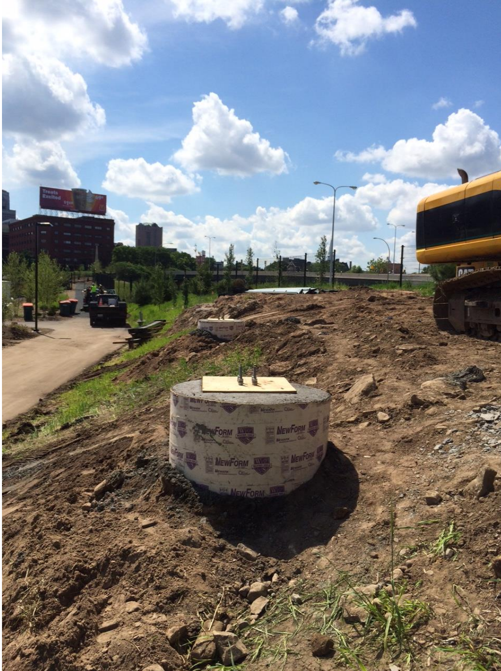
Image 1. Northeast array foundations; June 18, 2015
