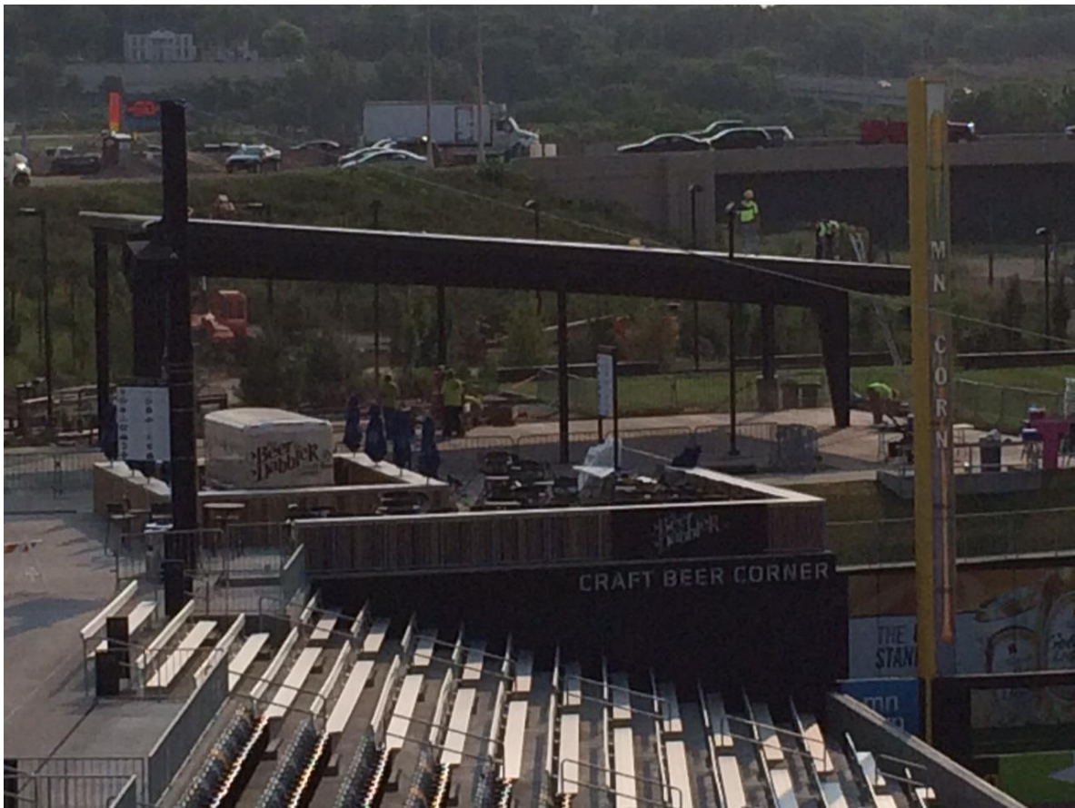
Image 6. Pavilion array construction progress; July 2, 2015
