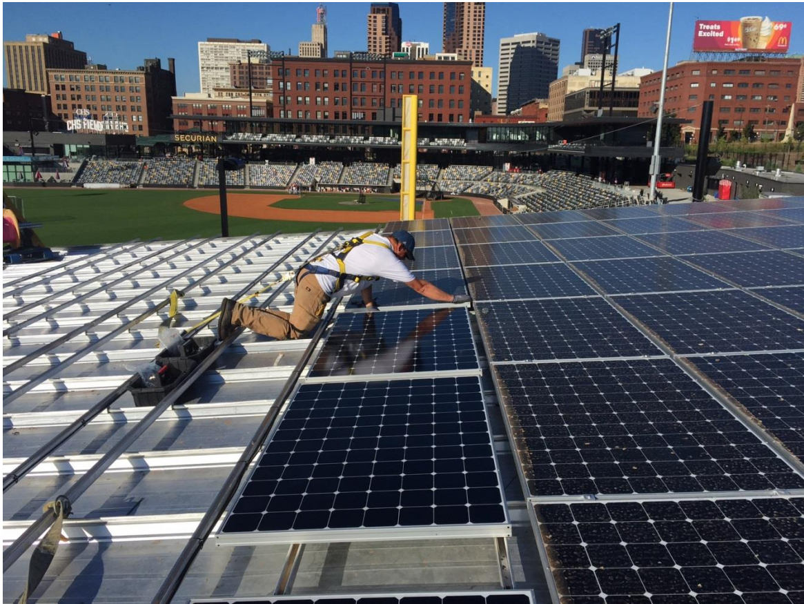
Image 9. Pavilion array solar panel installation; August 10, 2015
