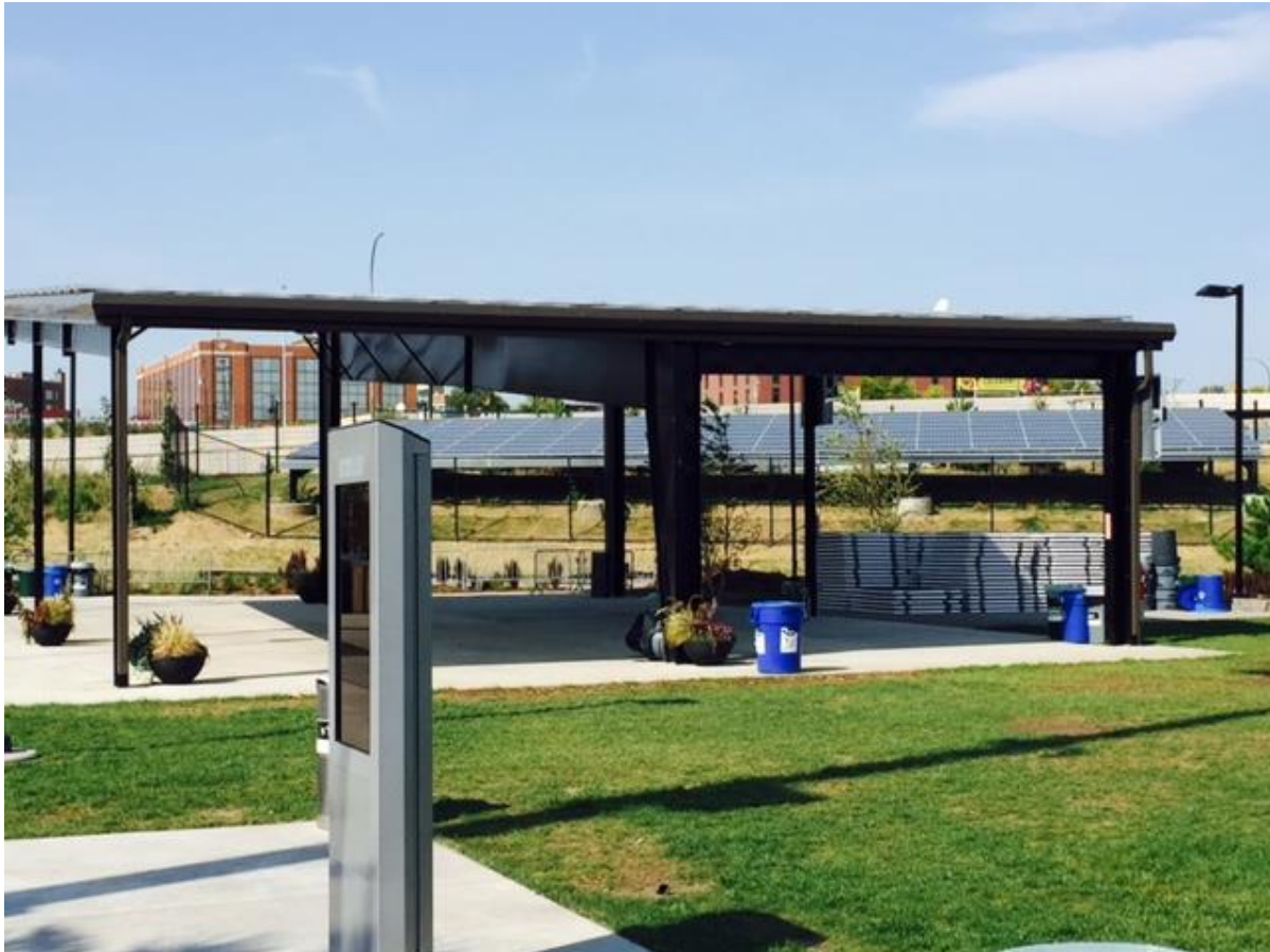
Image 11. Completed pavilion solar array with interactive kiosk in the foreground; September 9, 2015
