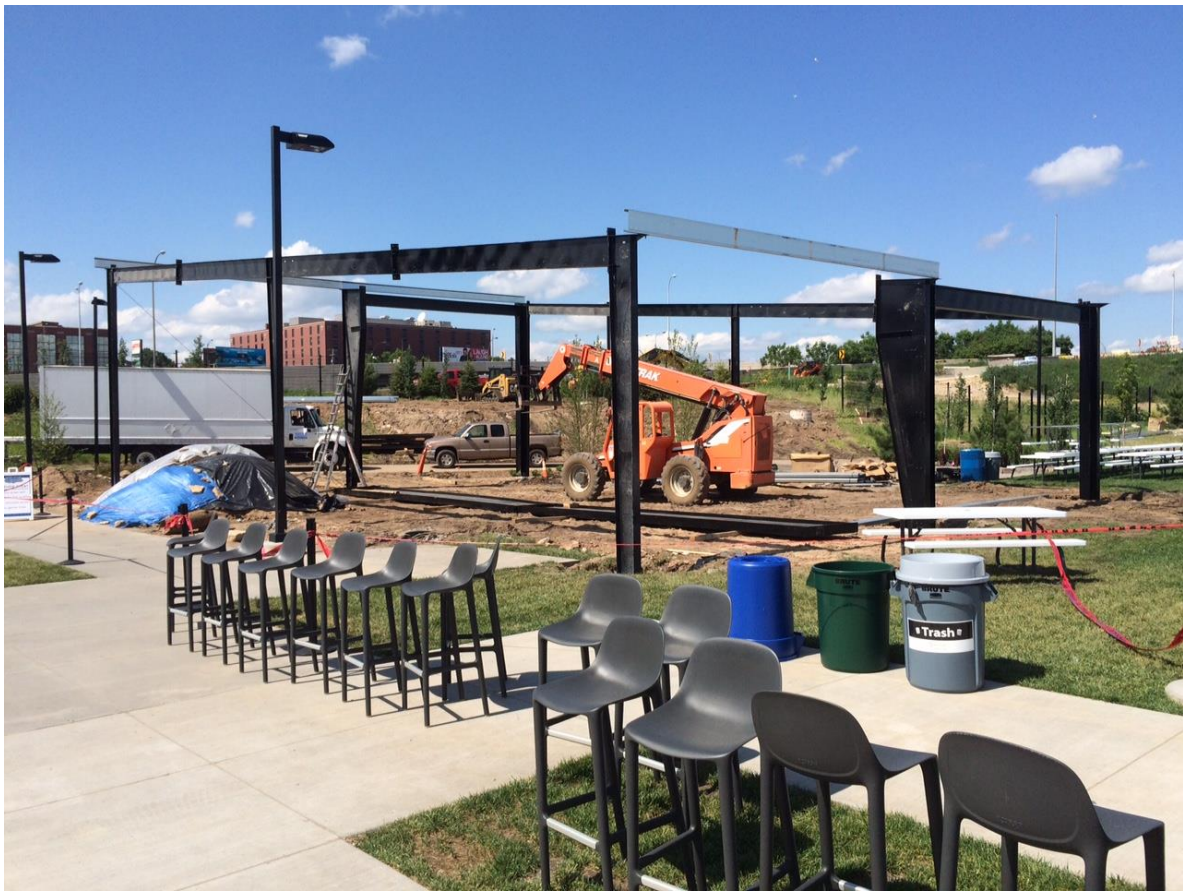
Image 2. Pavilion array steel construction; June 18, 2015
