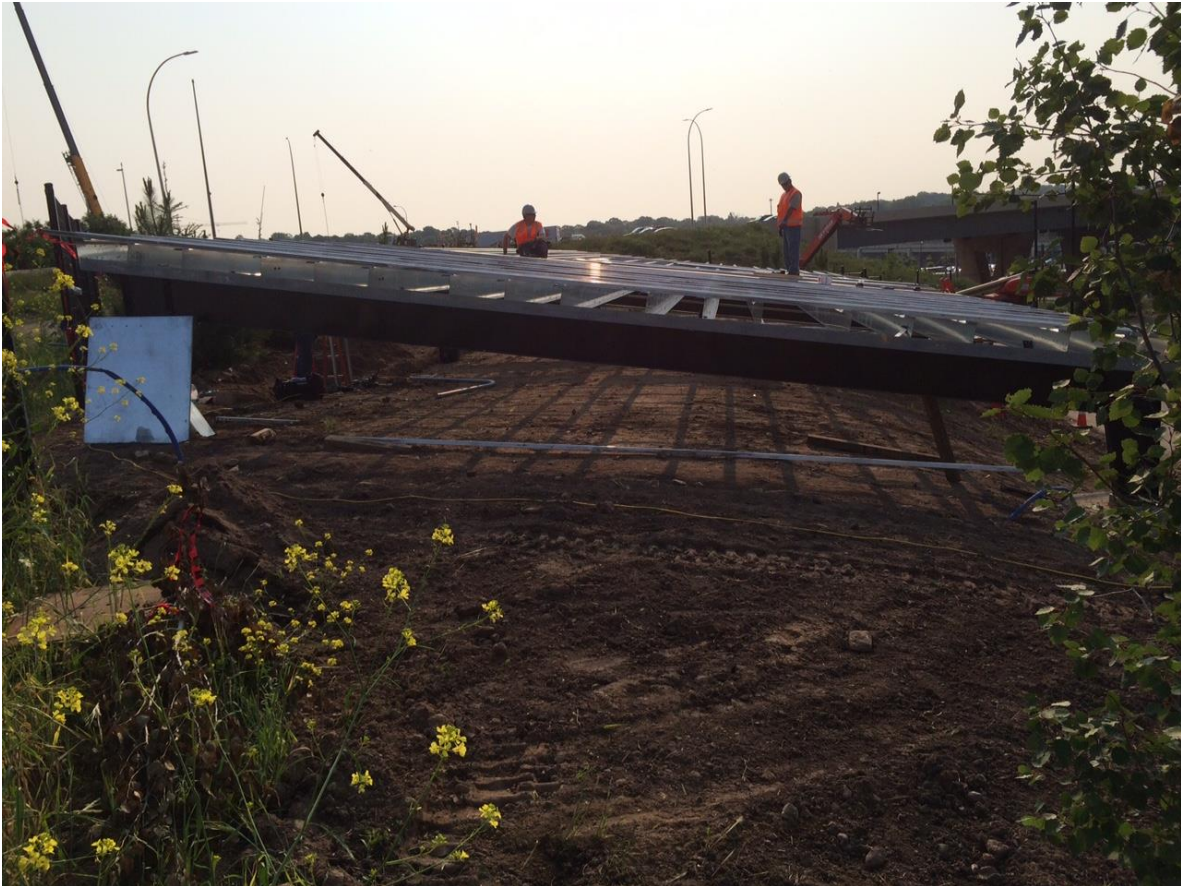
Image 5. Northeast array construction progress; July 2, 2015
