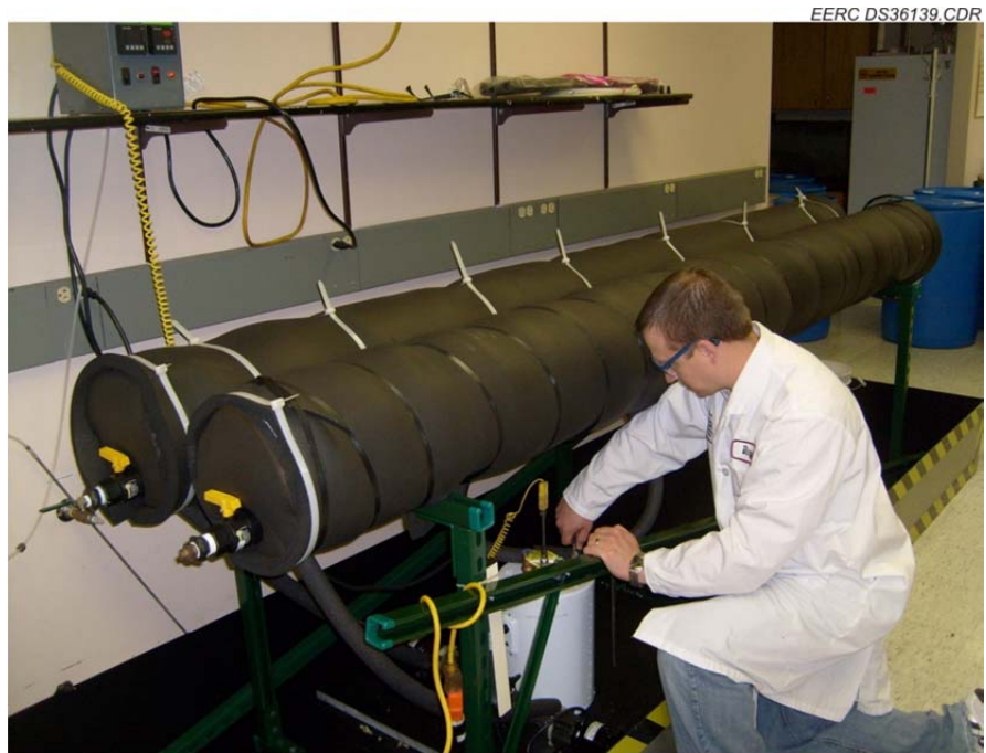
Figure 23. Closed-cell foam-insulated digesters.
